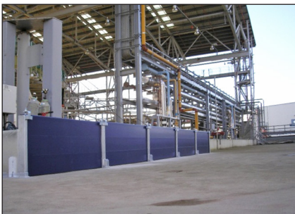
Multi-span 900mm high removable containment barrier.
