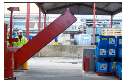
Gas-lift pivot barrier for vehicle access.
